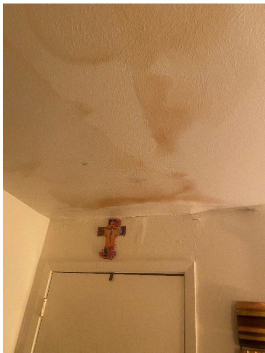
Photograph of Water-Stained Ceiling
