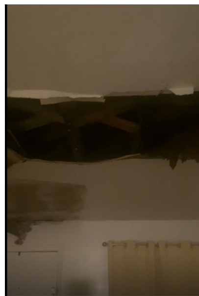
Image of Collapsed Ceiling
