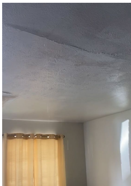
Image of Water Streaming from Ceiling (above the buckets in previous image)
