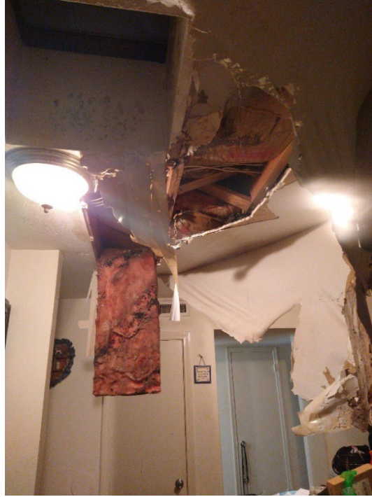
Photograph of Collapsed Kitchen Ceiling
